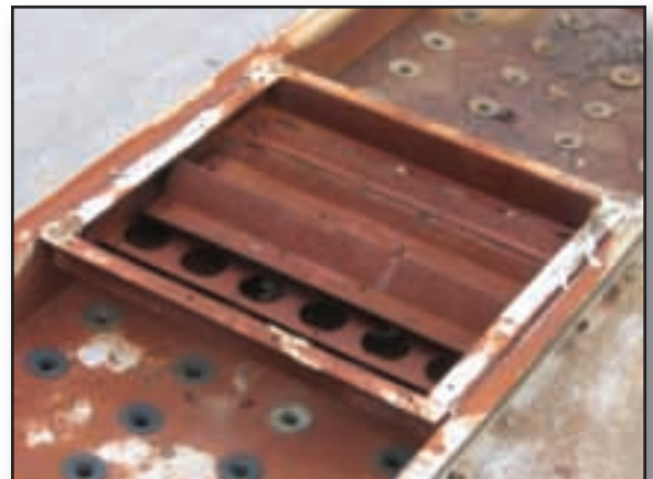
Corroded Hot Water Basin
