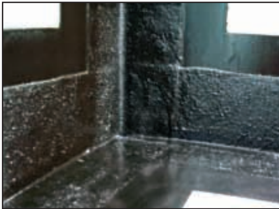
Extra Protection for Leaking Seams
