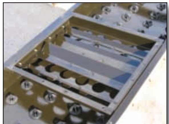
Hot Water Basin Coated with EvapLiner
